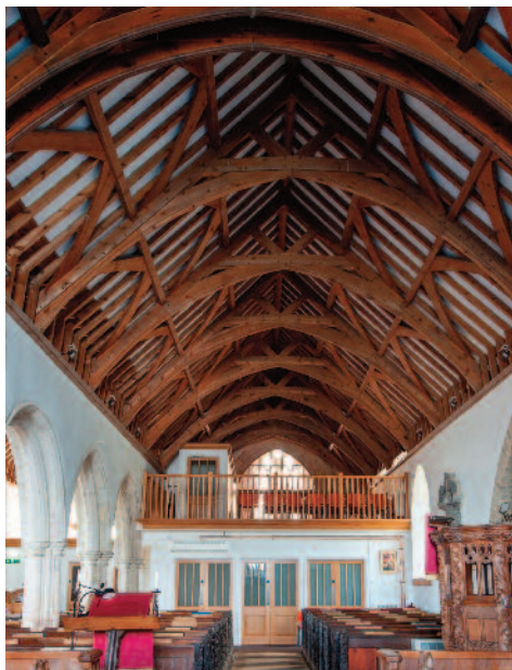
Gorran Church roof, a good example of J P St Aubyn's work
